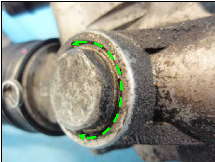
Inspect where noted.
